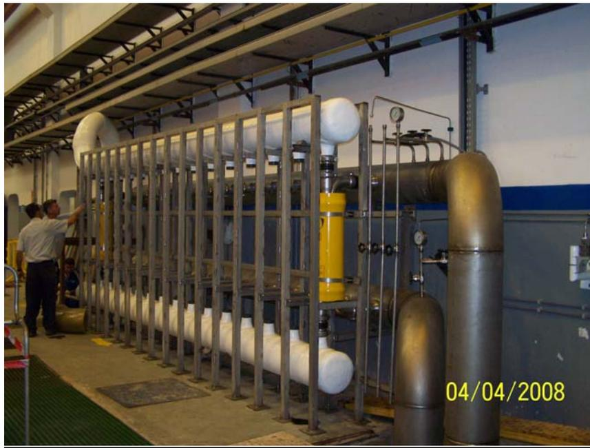
*Fig. 9. Installation of the pressure exchangers.*
